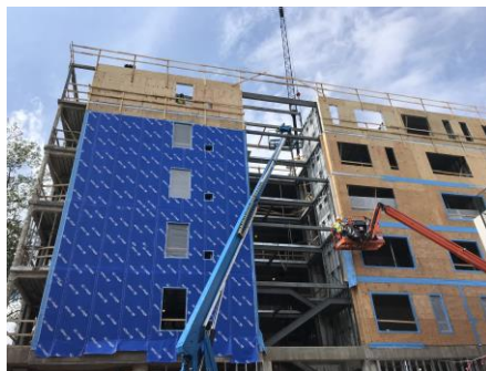
Air barrier installation
