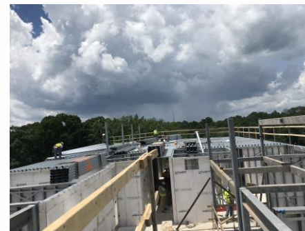
Roof deck prep
