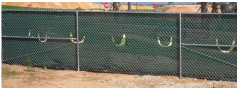
Construction LOD Fence
